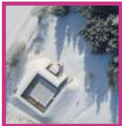
radar wind profiler
